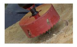
Pull the saw out of the cut keeping the drill bit in the hole it created, align your saw to be parallel with the roof slope, begin cutting and cut out a hole. Remove the plug lodged in the hole saw. As shown in image the top angle is correct. The step below will correct the bottom angle so the pipe will fit vertically.
