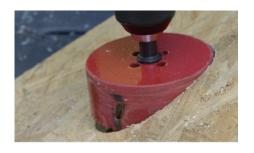
Align the outside wall of the hole saw with the first plumb cut you made, begin drilling doing your best to keep the saw plumb.
