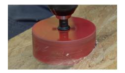
Place the drill bit of the hole saw in the center of the area of the penetration. Drill bit should go past the hole saw to penetrate deck. (do your best to keep the hole saw plumb)
