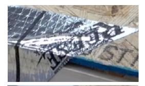
Place 6" or 9" flashing tape along the eave before the drip cap is installed. The flashing tape should extend down the fascia trim far enough to cover any gaps, but not so far that it will show beneath the drip cap.
