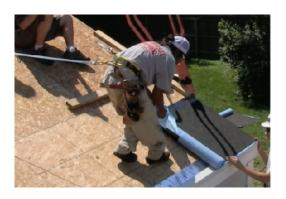
Stick a self-adhering membrane over the drip cap and onto the bare roof deck. Underlayment should be lapped at least 6 inches over the self-adhered membrane and continue up the roof.
